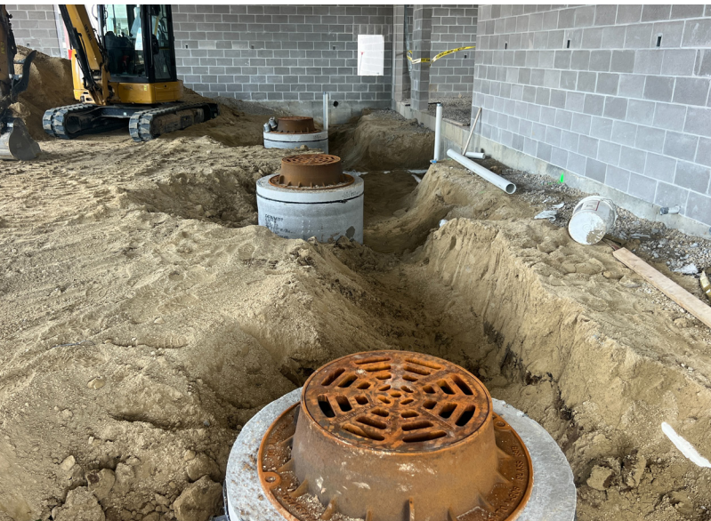
SETTING UNDERGROUND PLUMBING UNIT C
