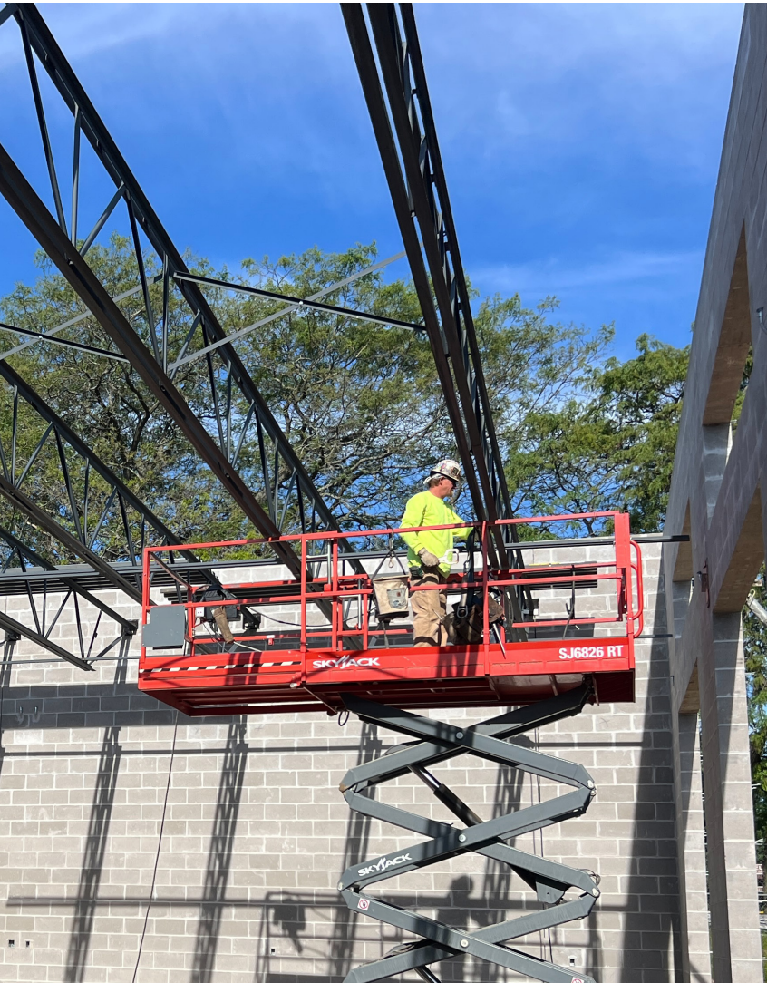
INSTALLING UNIT C ROOF JOISTS
